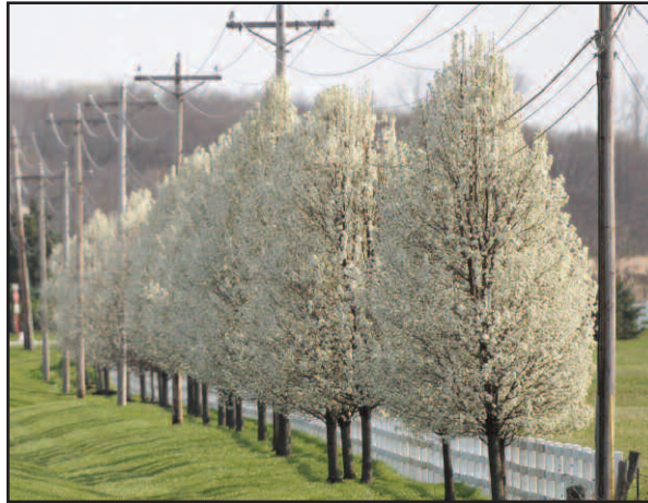
The property developer wasn't concerned with tree placement, but the local co-op will soon have to trim these trees to prevent a service disruption.
