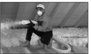
Heat flow resistance is measured or rated in terms of its R-value. The higher the R-value, the greater the insulation's effectiveness. When calculating the R-value of a multilay-
